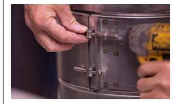
3. Place outer band around both sections covering the space between the shells. The flanges on the outer band fit into the grooves on the shells. Use a 3/8" nut driver to tighten into place.
